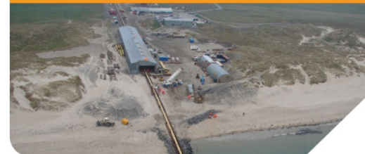
Wick Fabrication Site, UK
