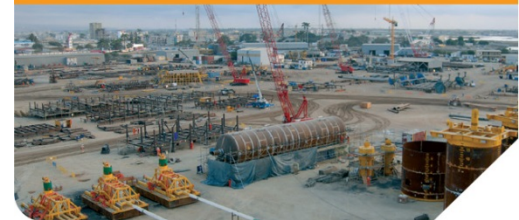
Lobito Fabrication Site, Angola
